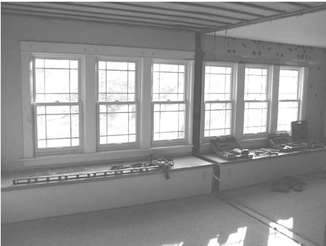
The wall between the two rooms has been removed and two new headers have been installed to carry the weight of the roof. The headers were made in two parts. One part runs east and west and replaces the previous wall that separated the two
