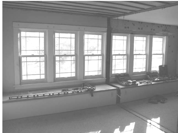
A view of the new library under construction.
