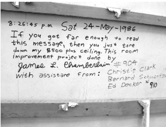
Archives uncovered during the building of the 3 rd floor library.
