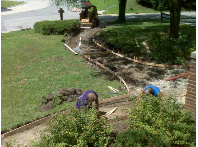
The picture shown below shows the new sidewalk after it has poured and set, and the forms removed. This is Brother Alex Moraniec - #1043 installing more soil and mulch around the new light pole and bushes that were planted at the intersection between the new sidewalk and parking sidewalk along the front of the chapter house.
