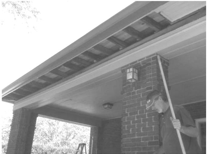
Work on replacing and painting the soffits was also completed in May. We were concerned that the rotted wood might extend up to the rafters holding up the roof over the porch. Fortunately, only a very few of the rafters suffered any damage, and the damage that was found was slight, so the work required to replace the soffits end up being significantly less than was feared.
